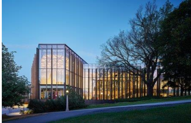
National Arts Centre Rejuvenation Ottawa, ON Diamond and Schmitt Architects Incorporated
