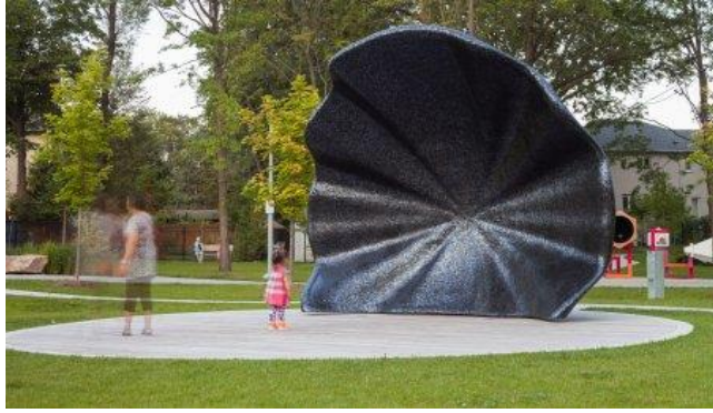
Limelight Bandshell North York, ON Paul Raff Studio Incorporated Architect
