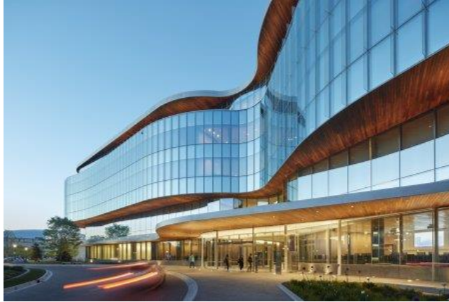
Kellogg School of Management, Northwestern University Evanston, IL, USA KPMB Architects
